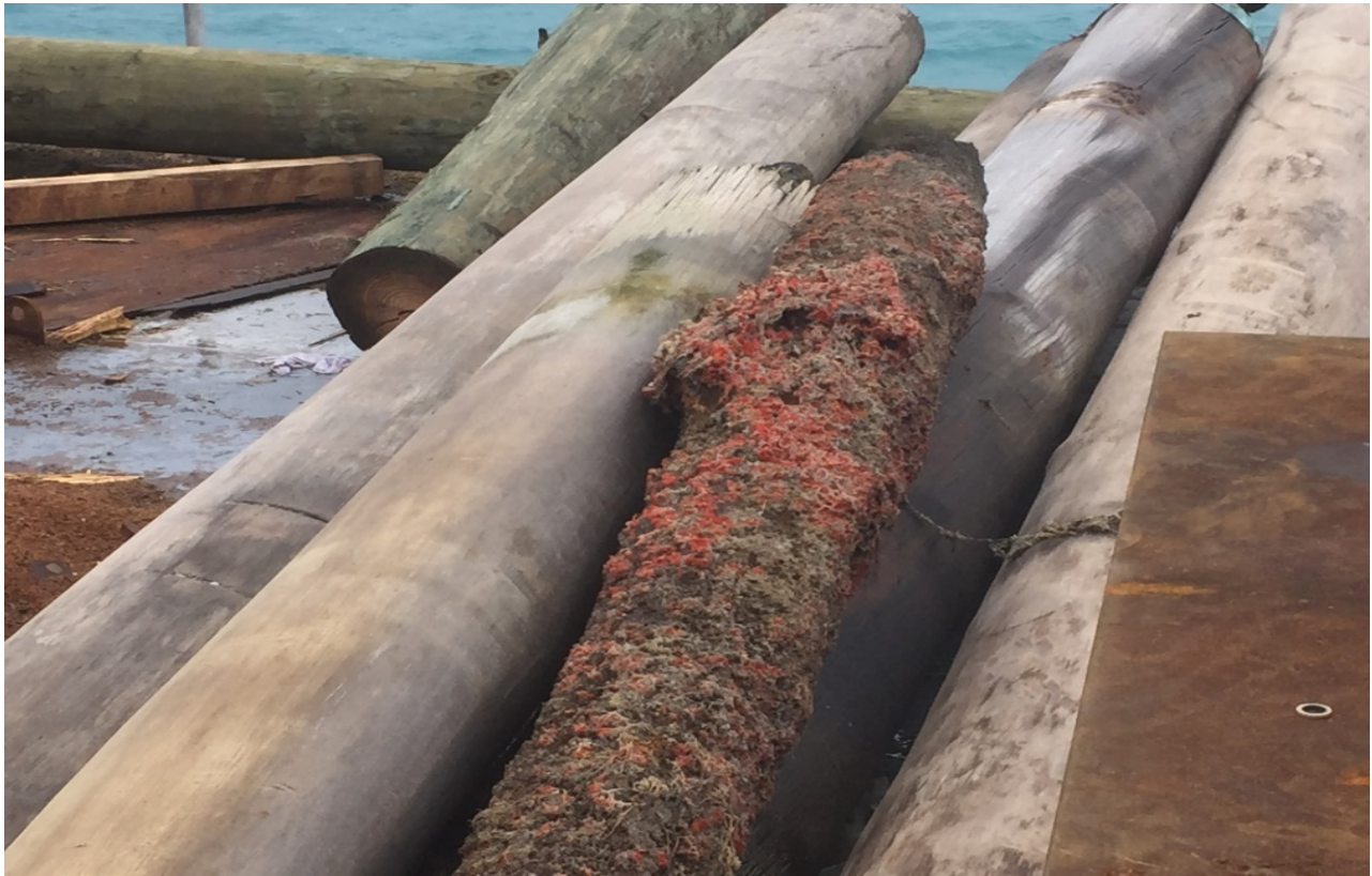
Completed Wood Piles Removal
