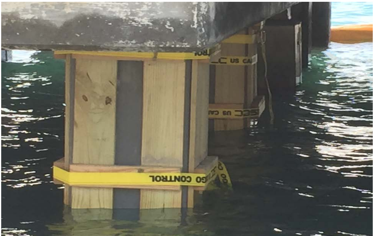
Reinforcement of Concrete Piles WIP
