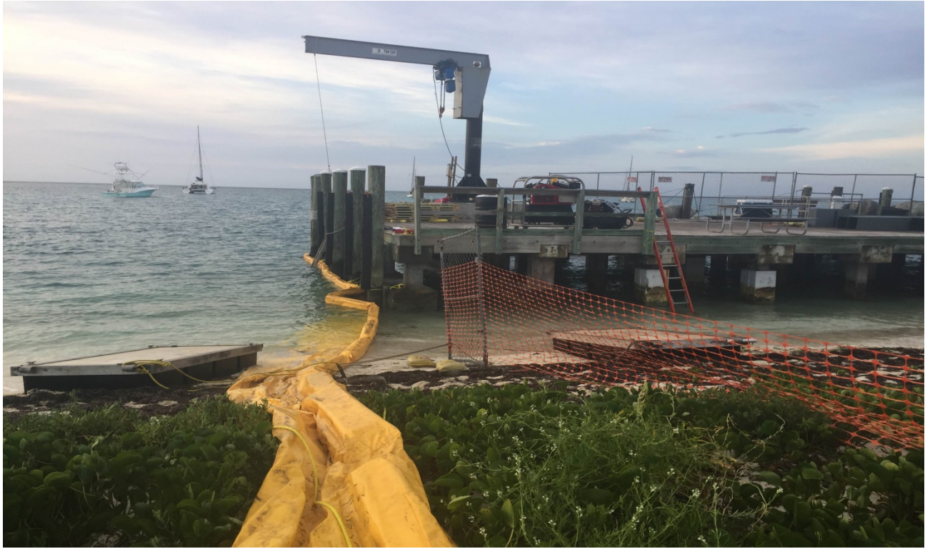
Equipment Set Up for Removal of Wood Piles
