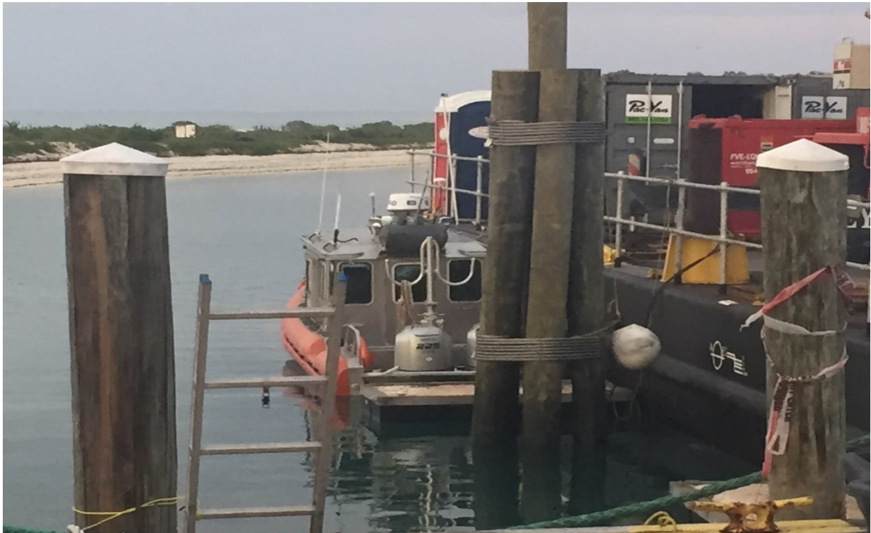
Removal of Wood Piles in Progress
