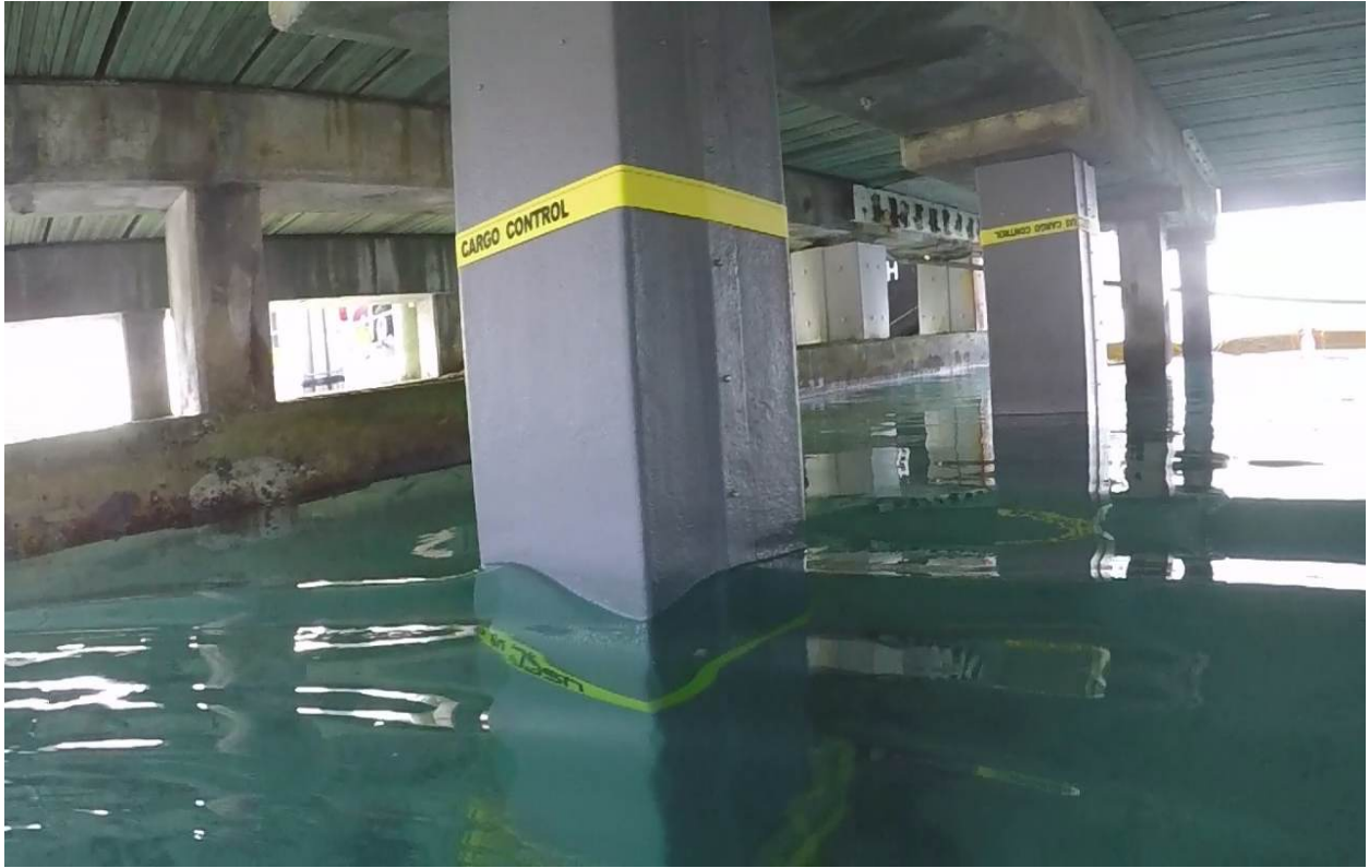
Completed Reinforcement of Concrete Piles
